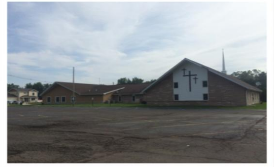
West Parking Lot
